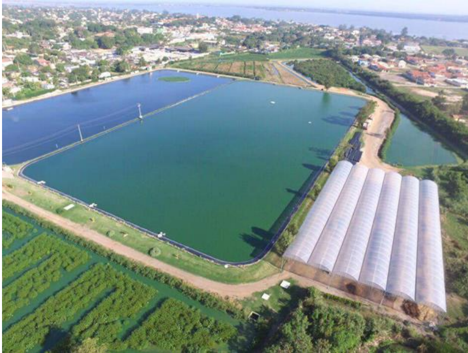
Figure 4. Current aerial view of ETE Ponte dos Leites.
